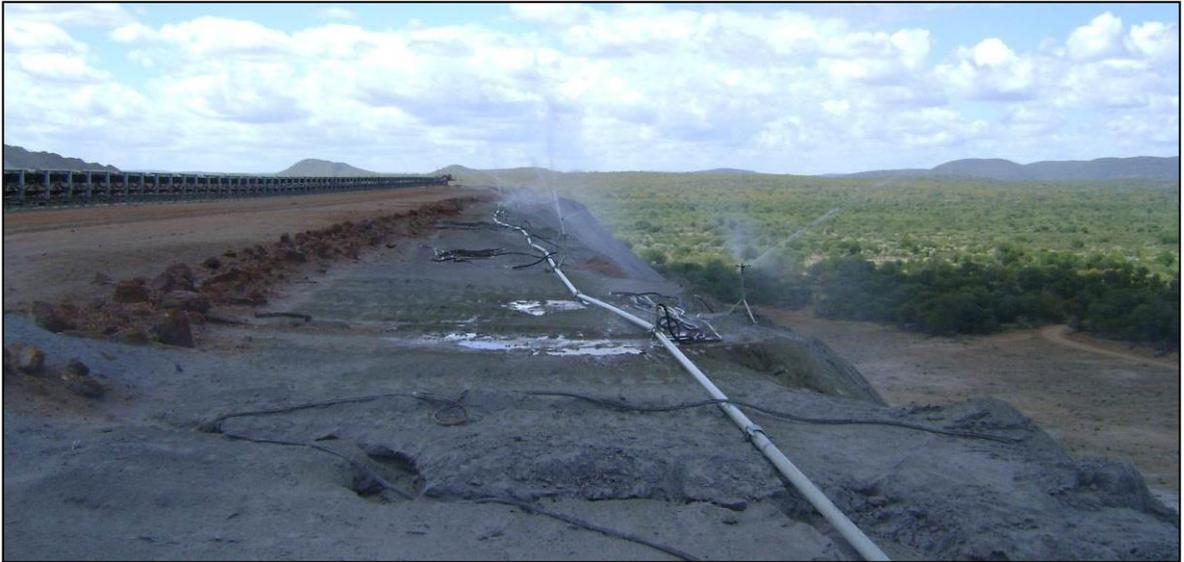
**Figure 12: Dust suppression system at Matimba Power Station**
